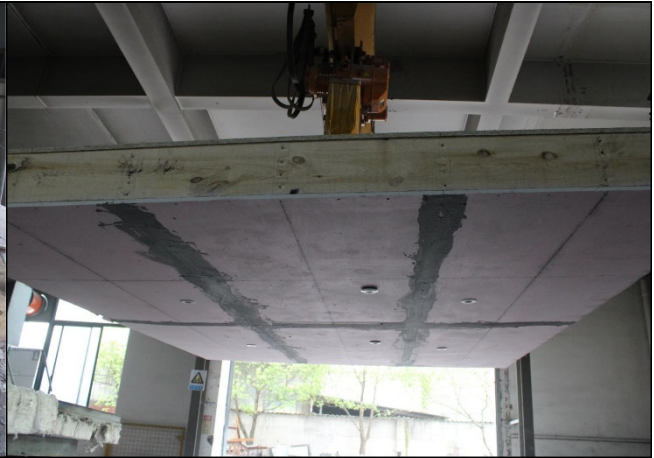
Photo 14: The exposed face before the test
